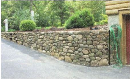
Figure 3-05. Retaining Wall Height
